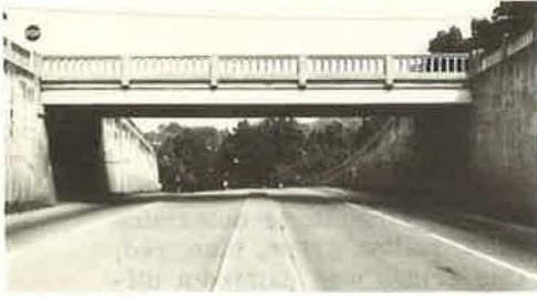
Figure 1. Locust Avenue bridge.
