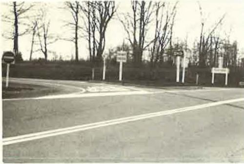
Figure 15. Suggested improvement on the exit ramp shown in Figure 14 by continuing the yellow lines and providing about a 24-in.-wide stop line. The island at the entry ramp is unnecessary.
