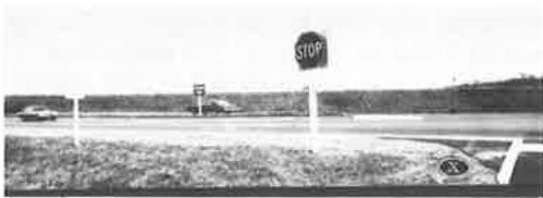
Figure 6. Suggested improvements on exit ramp and crossroad shown in Figure 5 by improving sight distance for left turns, providing intersection geometry sign at X, moving stop line closer to edge of crossroad, marking left corner flare, decreasing width of crossover, providing median nose delineators, and bringing signs on median closer to nose.
