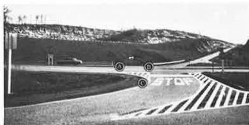
Figure 12. Suggested improvements of left lane shown in Figure 11 by channelizing left lane by marking or by providing physical barrier along ABC and reducing pavement width, providing stop line, continuing pavement edge line of crossroad across exit ramp, providing missing signs, and providing geometry sign shown in Figure 9(b).
