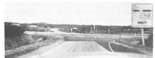
Figure 8. Suggested improvement on exit ramp shown in Figure 5 by use of intersection geometry sign.
