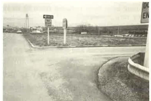
Figure 2. View from crossroad, with exit ramp on right, where wrong-way entry took place.
