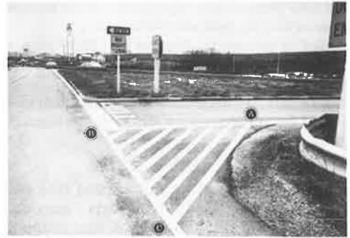
Figure 4. Suggested improvements of exit ramp shown in Figure 2 by marking pavement in flared corner and providing a very thick line—minimum of 24 in. (0.6 m)—with its outer edge in line with the pavement edge line.
