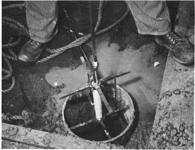
Figure 3. Installing strain meter and positioning bracket.
