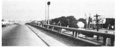
Figure 2. Flasher unit at overpass crest.
