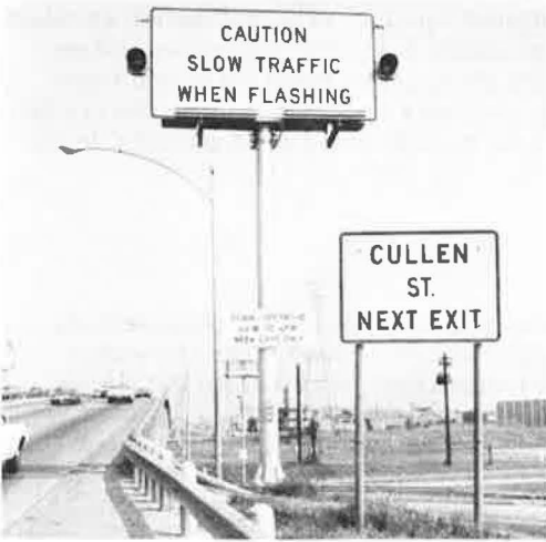
Figure 1. Warning sign with flashers.
