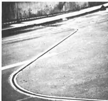
Figure 21. Unusually curved joint in Cologne-Bonn Airport upper departure level structure sealed with single-tube system.
