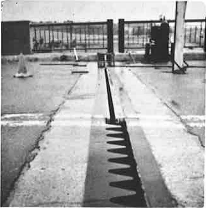
Figure 2. Seam-welded steel extrusion replacing old finger joint.
