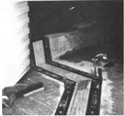
Figure 13. Factory-prefabricated unit incorporating vertical and horizontal bends.
