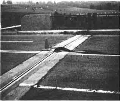
Figure 3. Installing strip seal element in one piece, a lane at a time, for 100 percent leakproofing.
