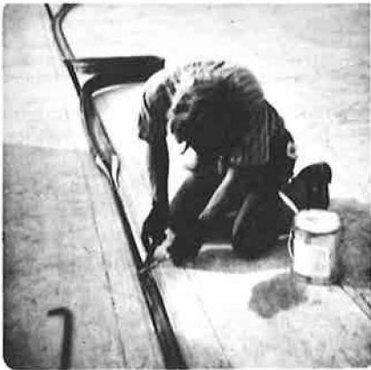
Figure 5. Field installation of strip seal gland.
