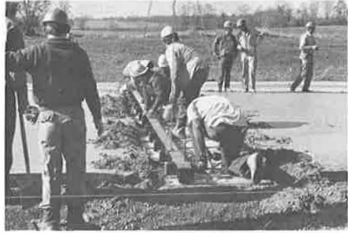
Figure 8. Placing female beam and bulkhead.
