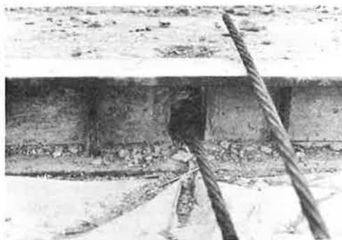
Figure 16. Anchor pocket in female beam.
