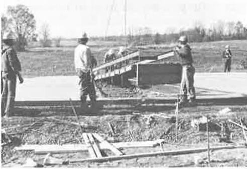
Figure 7. Lifting of blockout boxes.
