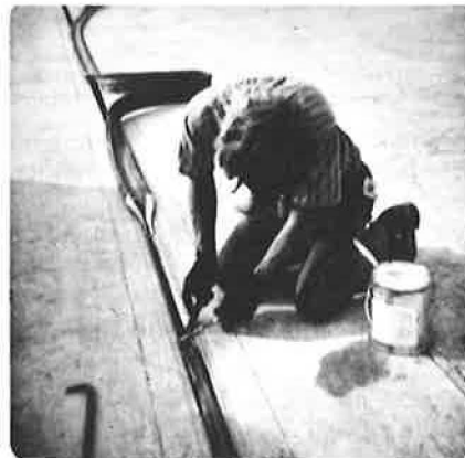
Figure 5. Field installation of strip seal gland.
