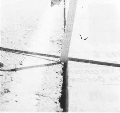
Figure 21. Trough formed between concrete pavement and asphalt shoulder.
