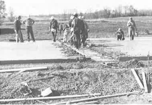
Figure 9. Placing concrete at joints.
