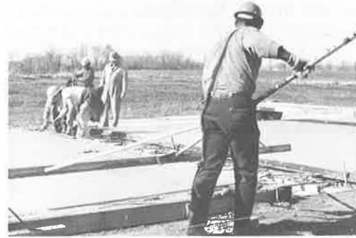
Figure 10. Finishing concrete at joint.
