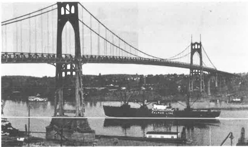
Figure 24. St. John's Bridge in Portland, Oregon, received new expansion joints.
