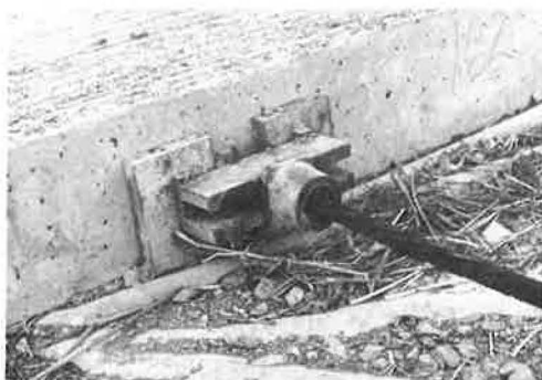
Figure 14. Jacking bridge.
