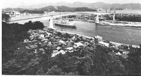
Figure 15. Urato Bay Bridge at Kochi, Japan, incorporates modular system at main-span joint.
