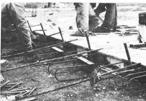
Figure 17. Placing male beams.
