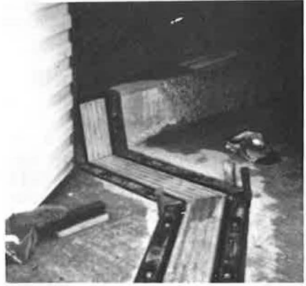
Figure 13. Factory-prefabricated unit incorporating vertical and horizontal bends.
