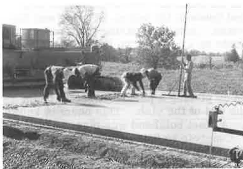
Figure 5. Preparing lifting ropes.
