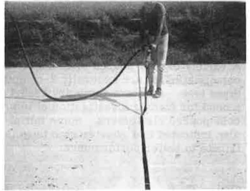
Figure 2. Sealing joint with rubberized asphalt.
