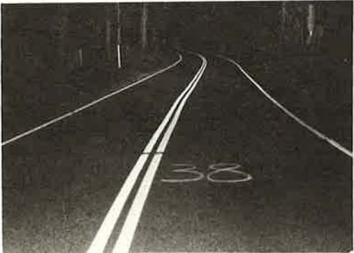
Figure 22. Test section 38, dry, April 27, 1974.
