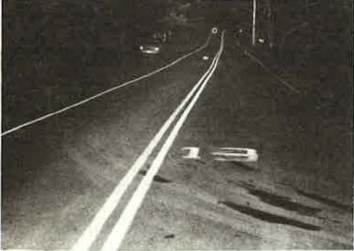
Figure 20. Test section 13, dry, November 6, 1972.
