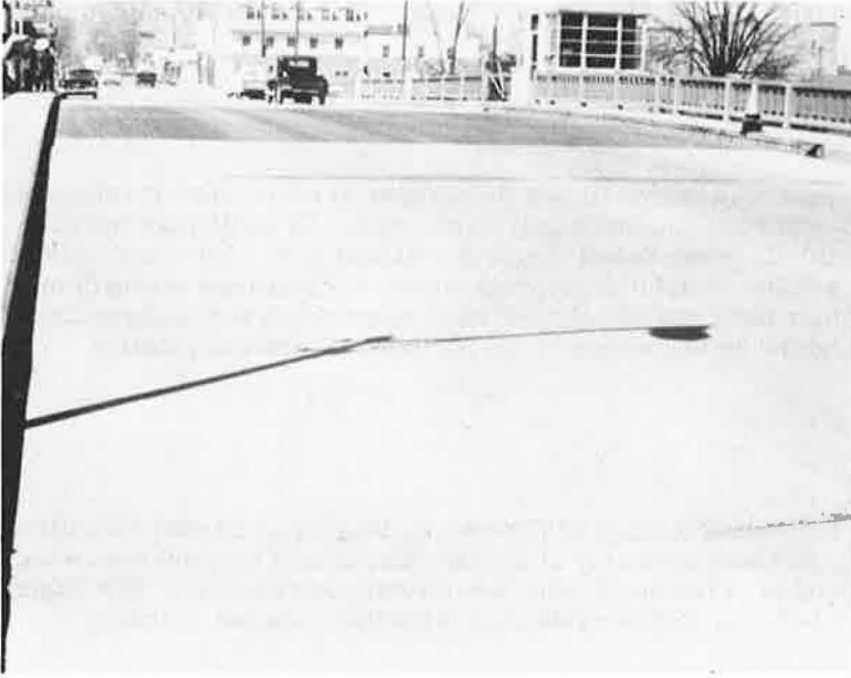
Figure 5. Mortar bridge surface after 13 years of service.
