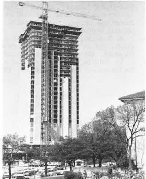
Figure 7. Architectural panels in place.
