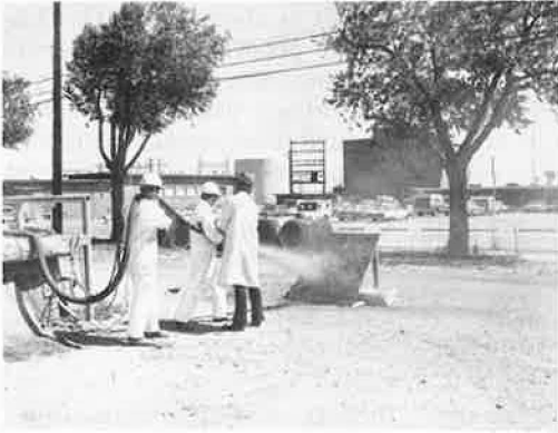
Figure 1. Application of polymer shotcrete using a modified commercial shotcrete gun.
