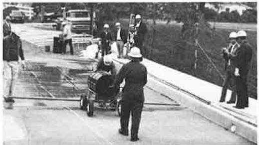
Figure 6. Applying monomer to concrete bridge deck.
