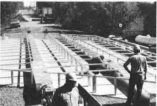
Figure 5. Drying one lane of small concrete bridge before surface impregnation.
