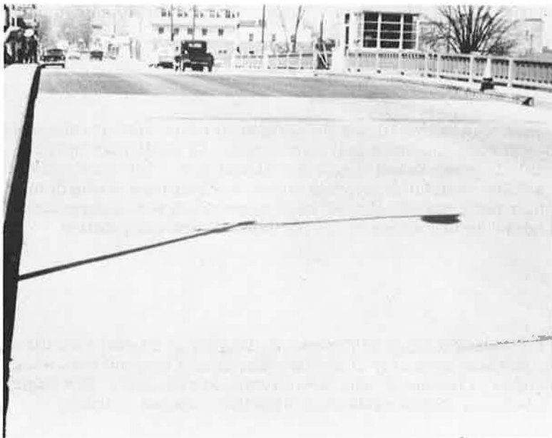
Figure 5. Mortar bridge surface after 13 years of service.
