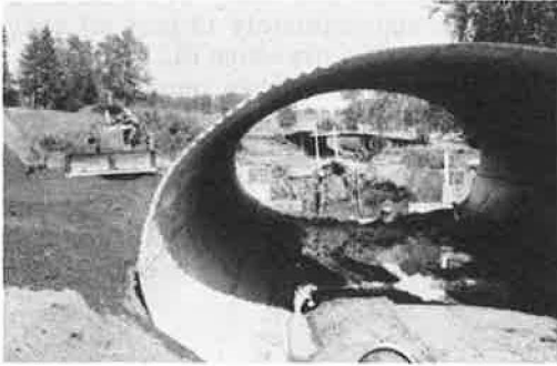
Figure 1. Structure under construction when backfill up to spring line.
