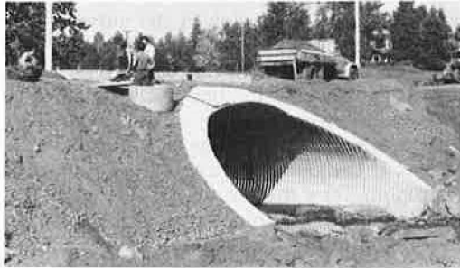
Figure 2. End view of completed structure with test load truck, readout station, and relief slab.
