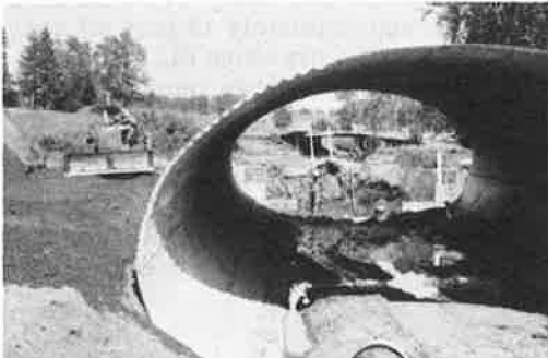
Figure 1. Structure under construction when backfill up to spring line.
