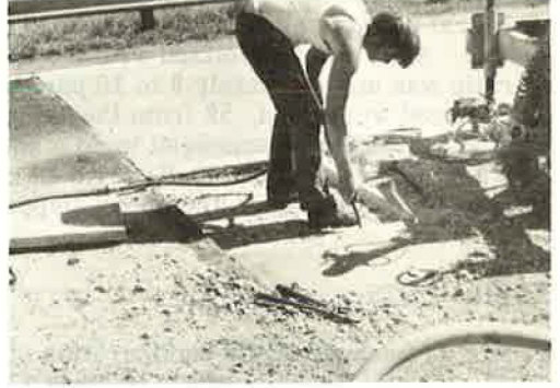
Figure 11. Steel mesh being removed from hole with hand tool.
