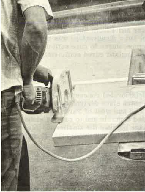
Figure 10. Precast slab being sawed to proper dimension.
