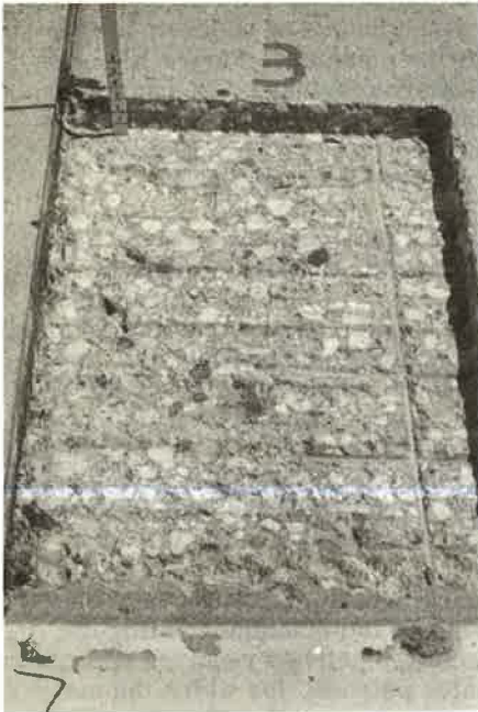
Figure 12. Grid pattern left after removal of steel mesh.
