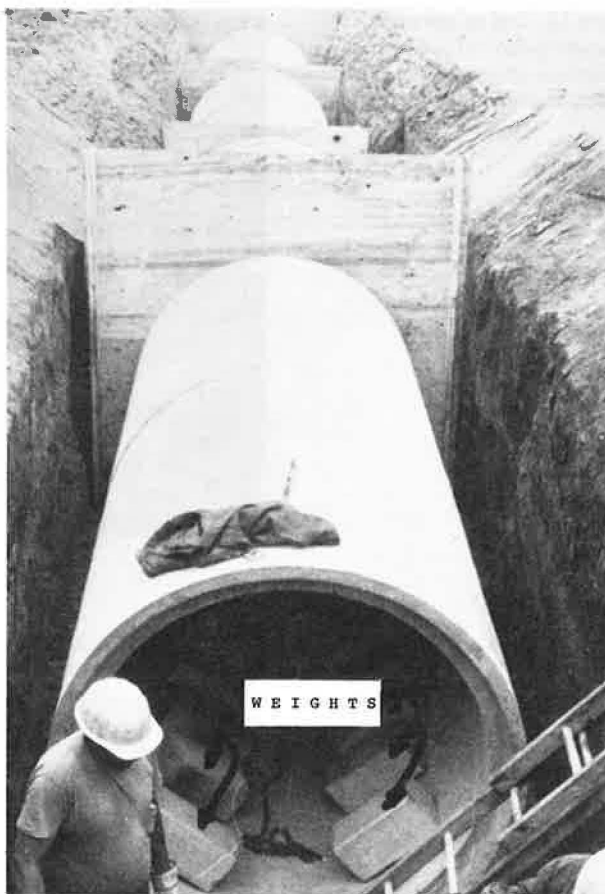
Figure 16. Phoenix test sections with bulkheads separating segments prior to backfilling.
