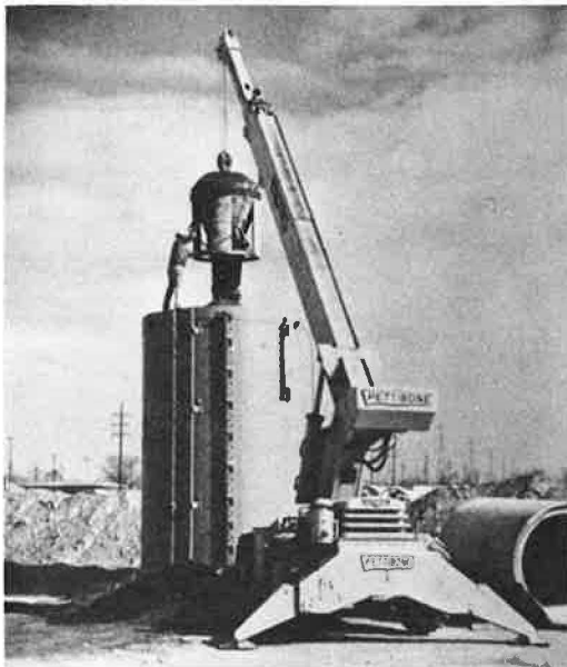
Figure 17. Sand being dropped into 126-in. (3200-mm) cylinder centered over alternate test sections to simulate field load.
