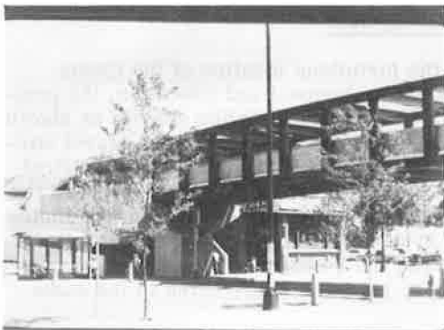
Figure 7. Pedestrian skyway over Cedar Avenue.
