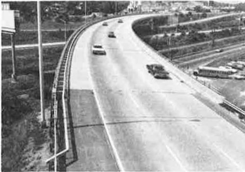
Figure 4. The completed system.
