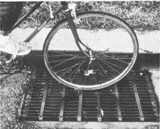
Figure 11. Street grate that is safe for bicycling.
