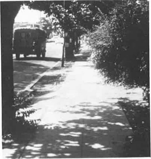
Figure 10. Sidewalk bikeway with inadequate clearance.
