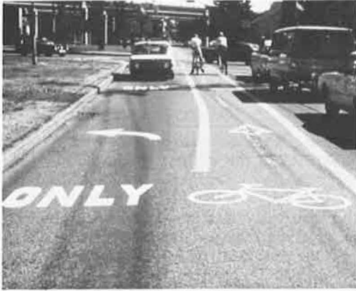
Figure 18. Placement of bicycle through lane between left and right automobile turning lanes in Seattle.
