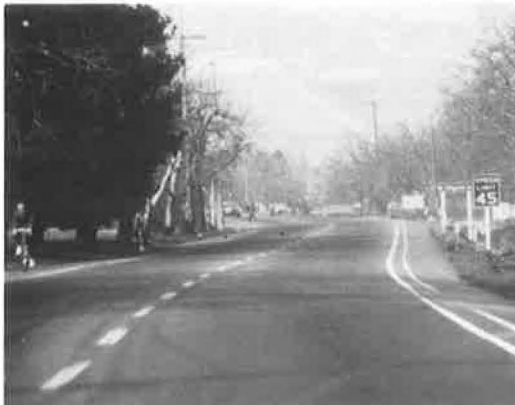
Figure 16. Exclusive bike lane on high-speed Danville Highway in California.
