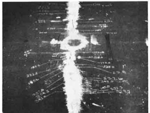
Figure 10. Reflection cracking pattern for symmetric loading.
