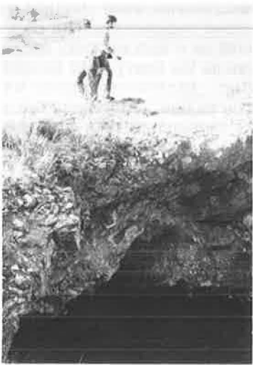
Figure 3. Collapsed ceiling rock over mine adjacent to survey line.
