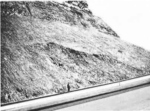
Figure 7. Small slide in cut slope at station 46 near Pacheco Pass.
