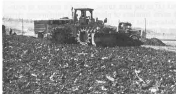
Figure 4. Sheepfoot compactor processing refuse-soil layer.
