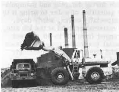
Figure 2. End loader breaking up hardened fly ash from stockpile.
