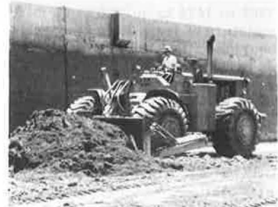
Figure 4. Blading fly ash in lifts.
