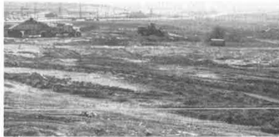
Figure 6. Bottom dump delivering load as rubber-tired bulldozer spreads soil over refuse.
