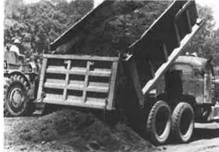
Figure 3. Spreading fly ash on grade.
