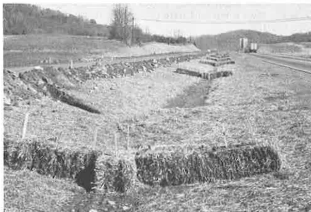
Figure 4. Experimental barriers in place.
