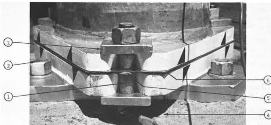
Figure 1. Slip base used with type 31 lighting standard in crash tests 311 and 312.
