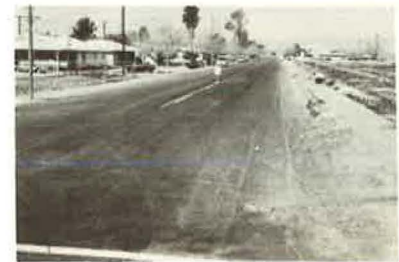
Figure 14. Asphalt-rubber seal coat placed directly on clay loam.
