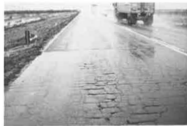
Figure 4. Asphalt-rubber seal coat on Aguila project in background.
