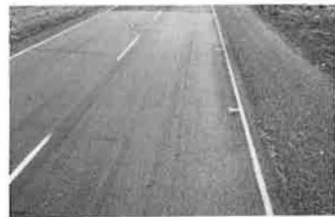
Figure 8. Minnetonka project after asphalt-rubber seal coat.
