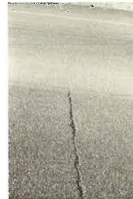
Figure 16. I-17 partially treated with asphalt-rubber.
