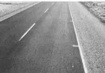
Figure 9. Minnetonka project after asphalt-rubber membrane interlayer.
