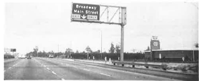
Figure 3. Typical EXIT ONLY treatment.
