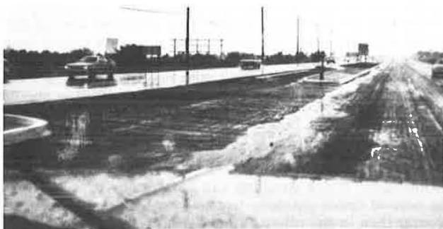
Figure 16. Unequal drainage properties.
