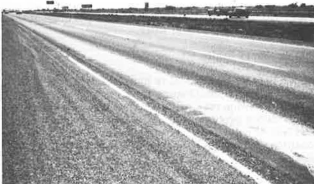
Figure 15. Maintenance crack patching.
