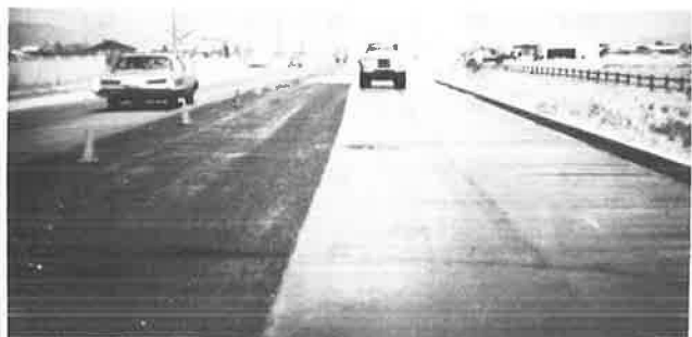
Figure 13. Chip or slurry seal occupying only a portion of a lane.
