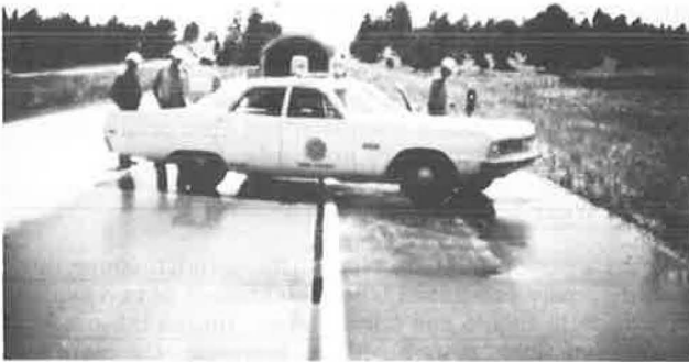
Figure 14. PCC pavement travel lane with AC distress lane.
