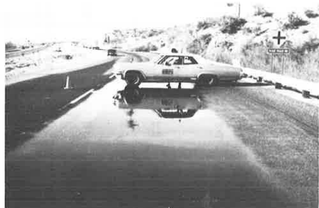
Figure 12. Differential flushing or bleeding.
