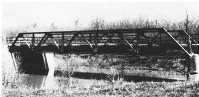
Figure 1. A typical pony truss bridge.
