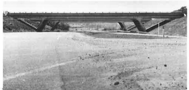
Figure 1. Test structure on I-64 over US-250 east of Charlottesville, Virginia.
