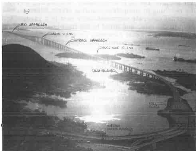
Figure 2. Northwest view of Rio-Niteroi bridge.
