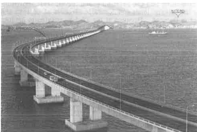
Figure 3. East view of Rio-Niteroi bridge.
