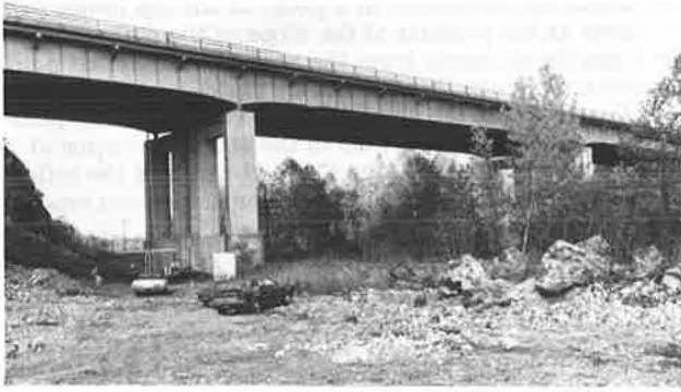
Figure 1. Lehigh Canal bridge (instrumentation installed in left side span).
