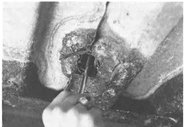
Figure 7. Corroded form and deteriorated concrete at location of foreign material in deck.
