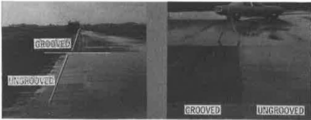
Figure 8. Water drainage from grooved and ungrooved asphalt. Grooving pattern, 38 x 6 x 6 mm (1-1/2 x 1/4 x 1/4 in.).
