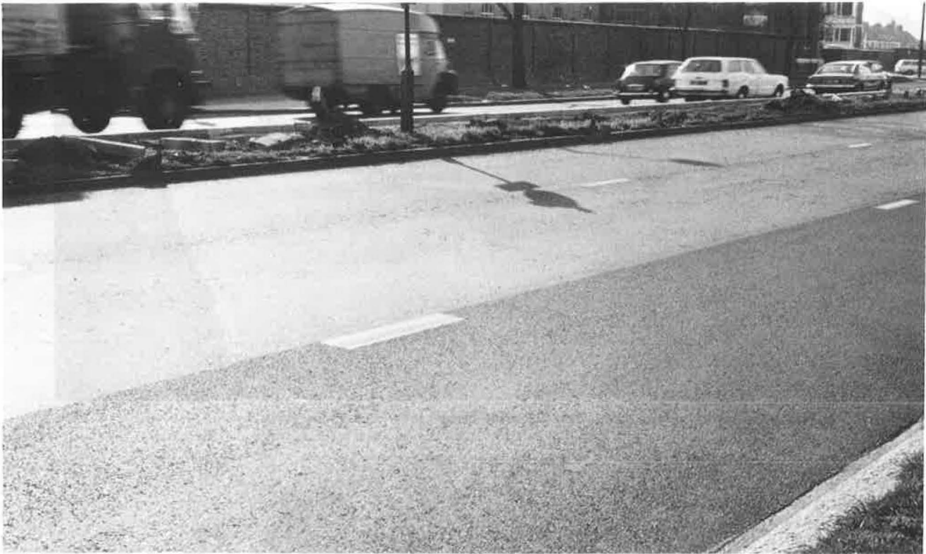
Figure 11 Epoxy friction course on A4 road, Hammersmith, after 2 years.
