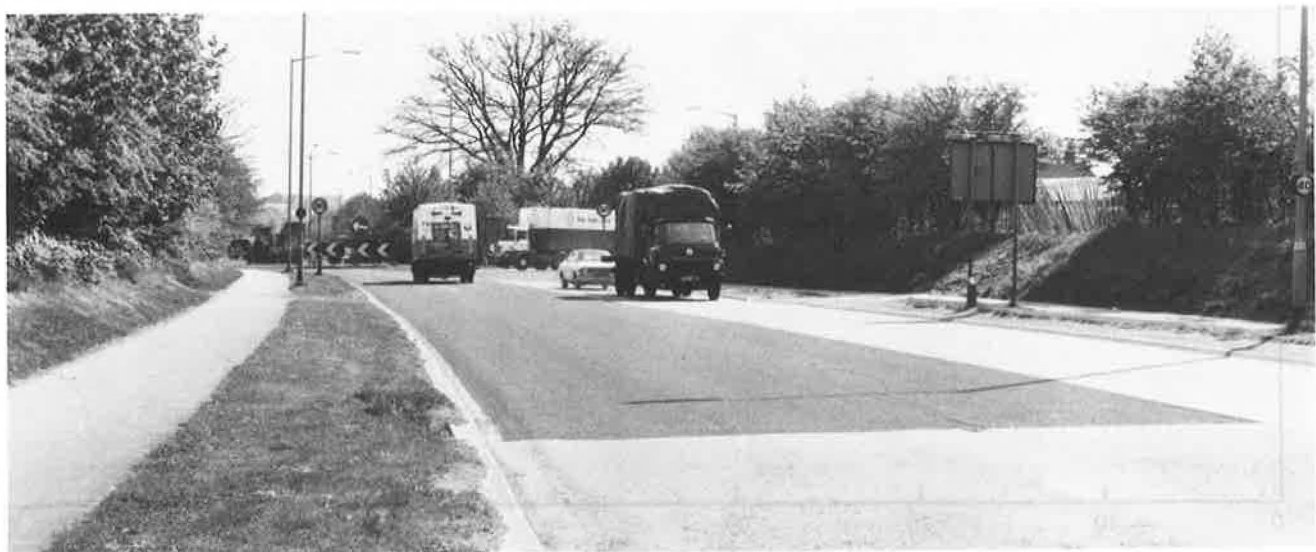
Figure 5 Shellgrip treatment on the approach to a roundabout on a high-speed road in England.
