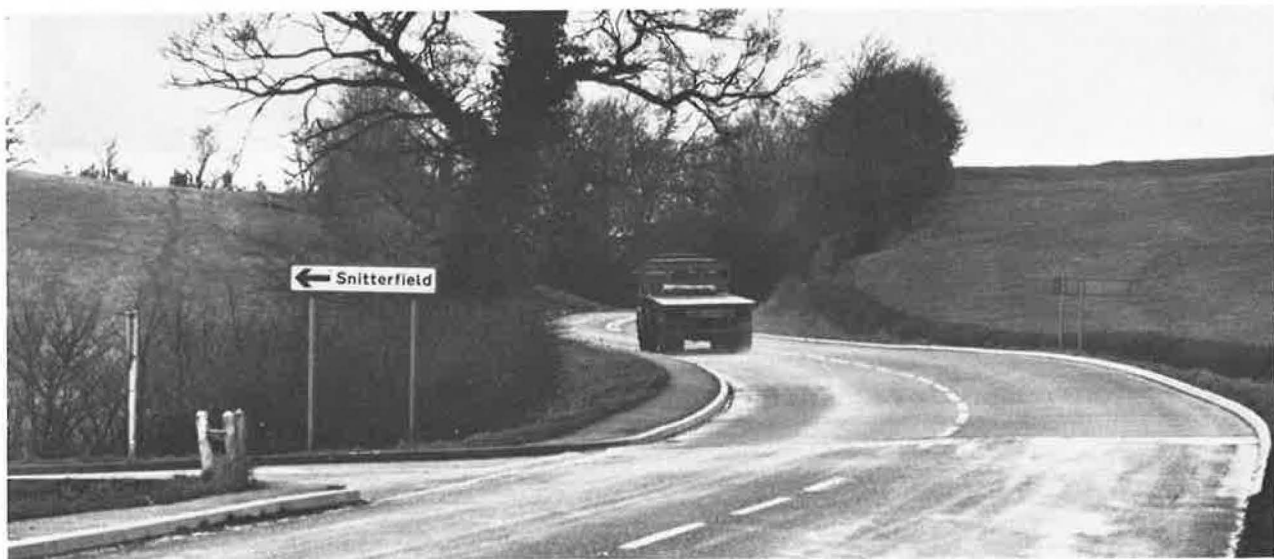
Figure 10 Same lorry on friction course with junction between the two surfaces clearly visible. (With acknowledgement to Mr. I.A. Cram, Warwickshire)
