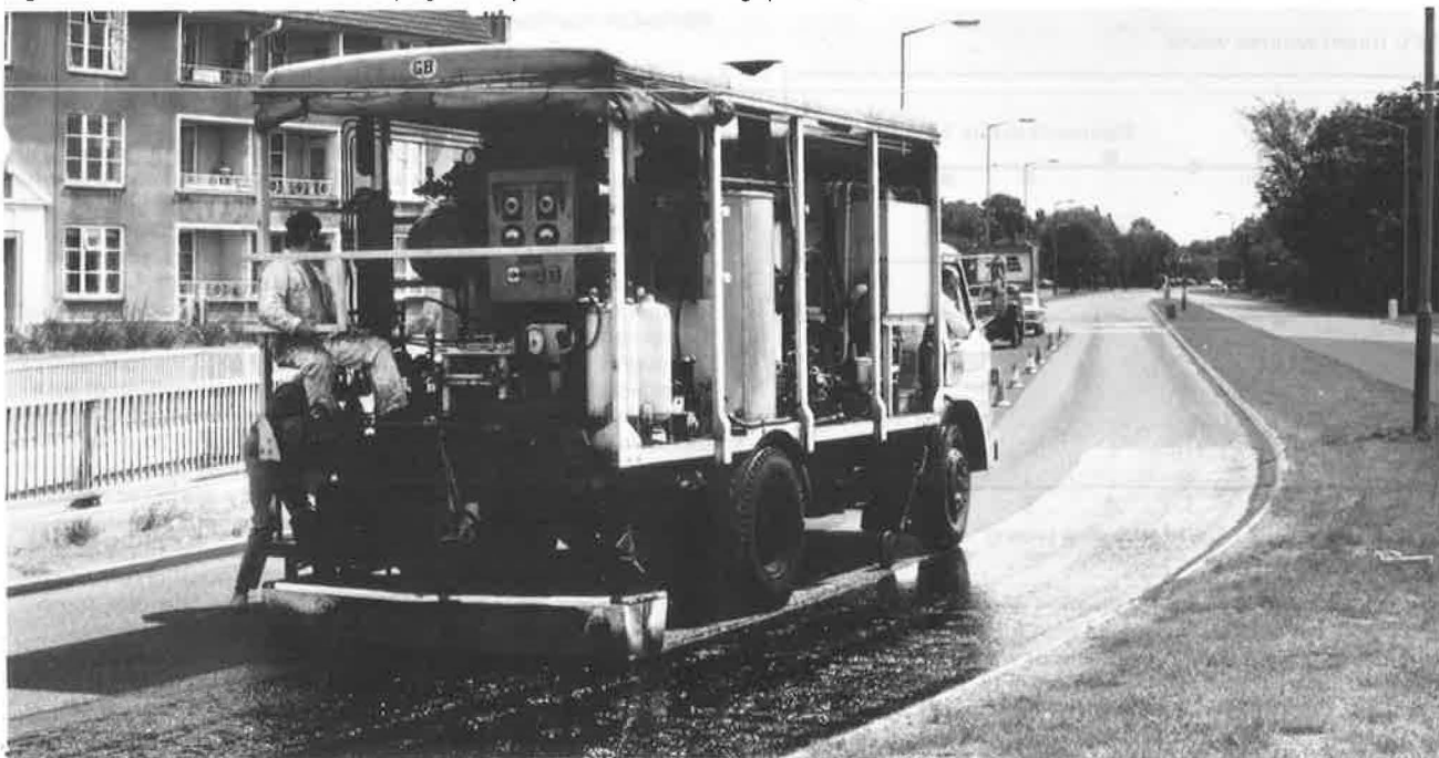
Figure 3 The Coleman machine laying two adjacent widths of Shellgrip binder.
