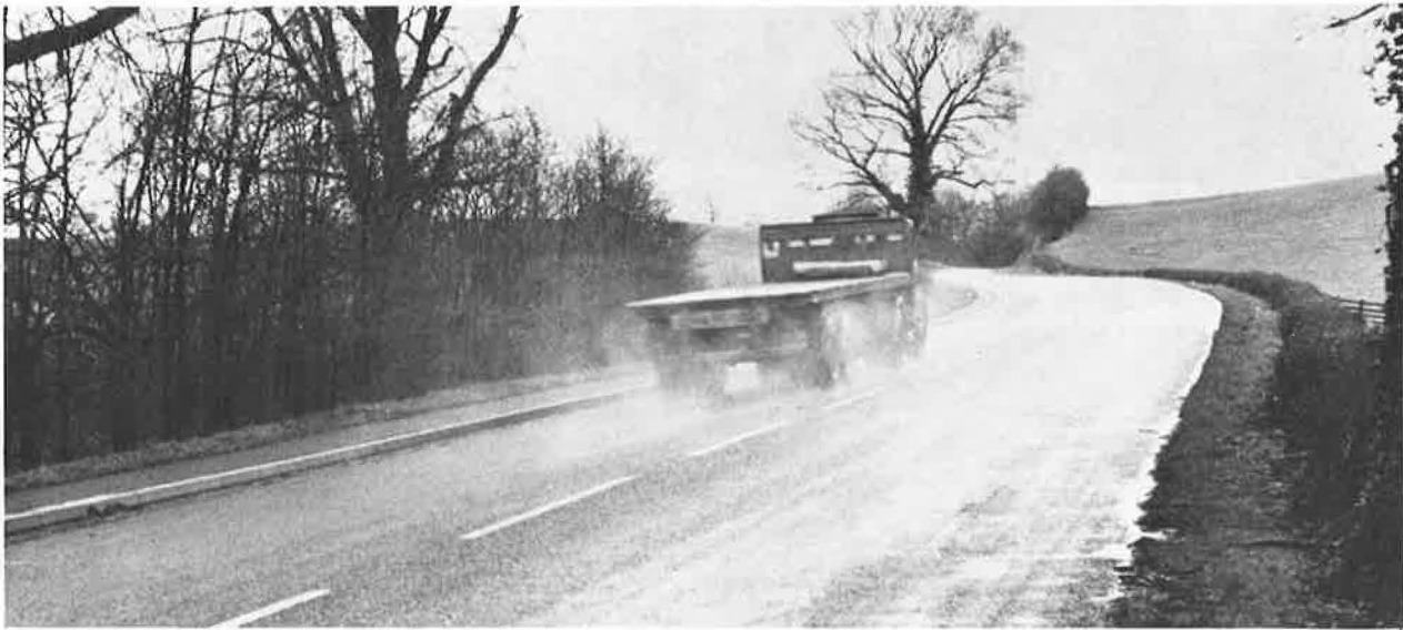
Figure 9 Lorry on typical impervious surface in rain. (With acknowledgement to Mr. I. A. Cram, Warwickshire)
