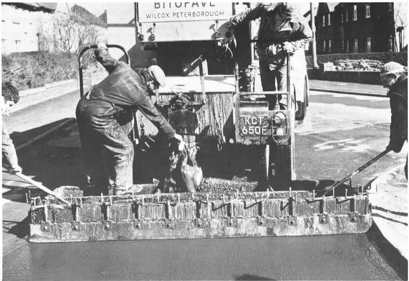
Figure 13 Slurry seal being laid on residential street.
