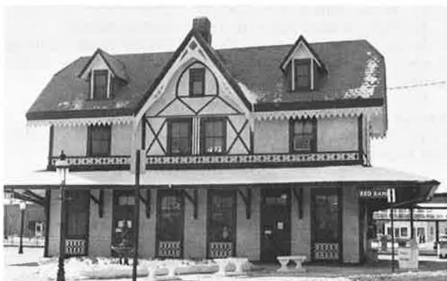
Figure 5. Red Bank Station after restoration (1976).
