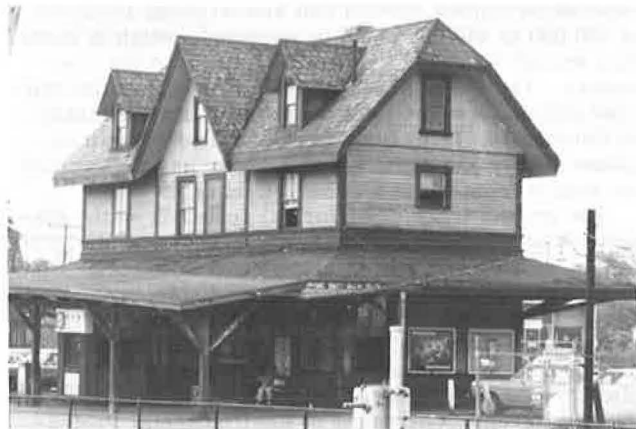
Figure 3. Existing station in May 1975.
