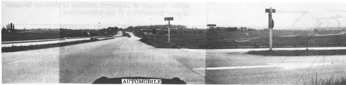
Figure 6. Daytime photograph of partial cloverleaf intersection of Interstate exit ramp and primary highway.
