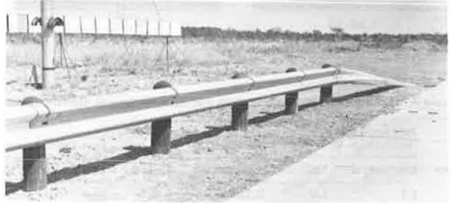
Figure 19. Guardrail and terminal before test 3.
