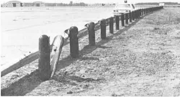
Figure 22. Position of vehicle and damage to guardrail after test 4.
