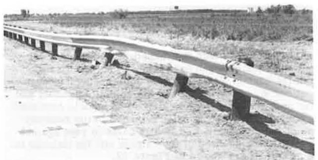
Figure 21. Guardrail after test 3.
