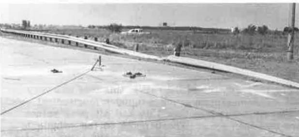
Figure 17. Guardrail and terminal after test 2.
