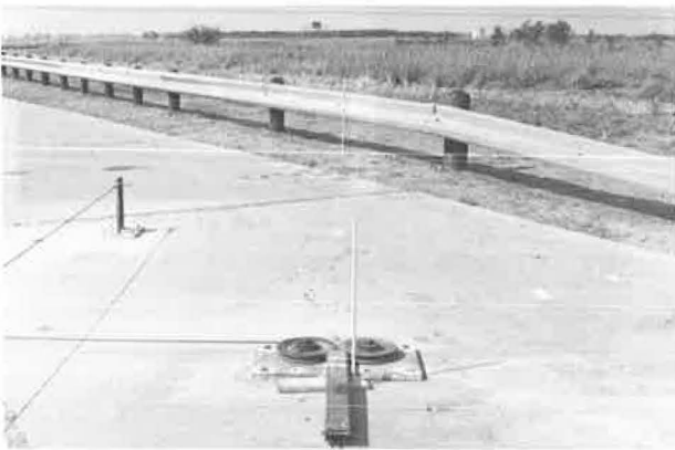
Figure 15. Guardrail and terminal before test 2.
