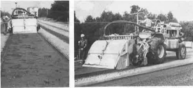
Figure 9. Pulverization by using a pulvimixer.
