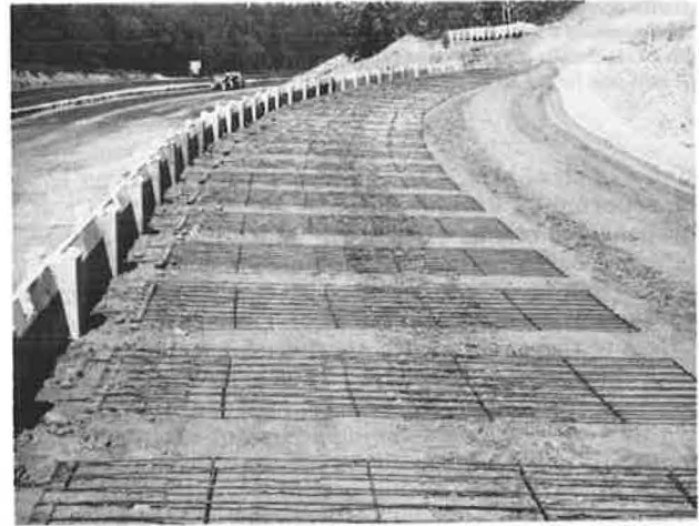
Figure 2. Bar-mesh reinforcement in mechanically stabilized embankment on I-5 at Dunsmuir, California.
