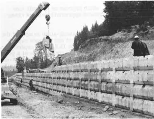
Figure 1. Concrete-beam facing of mechanically stabilized embankment on I-5 at Dunsmuir, California.
