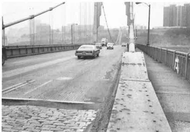
Figure 5. Tenth Street Bridge, built in 1932 (bridge 21).
