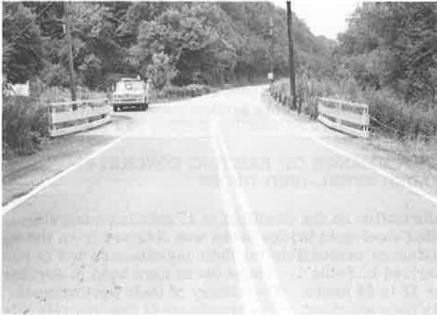
Figure 1. Concrete-filled steel-grid bridge deck built in 1934 (bridge 18).
