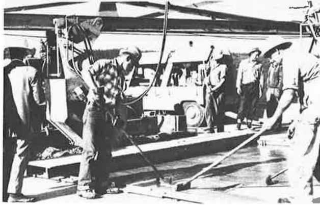
Figure 2. Paving the Port Mann Bridge.
