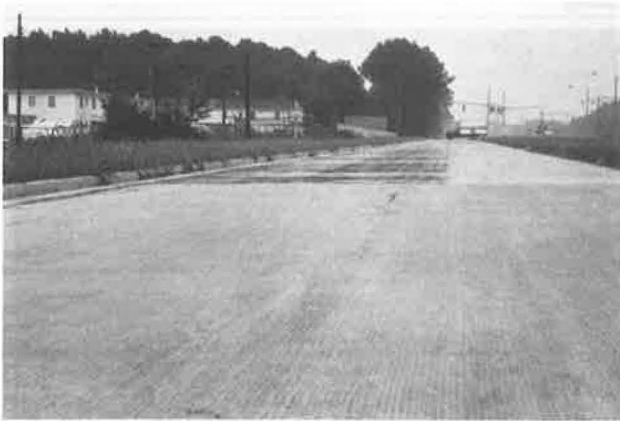
Figure 15. Contrast during rainfall between longitudinally and transversely tined texture (foreground) and conventional, longitudinally tined texture (background).
