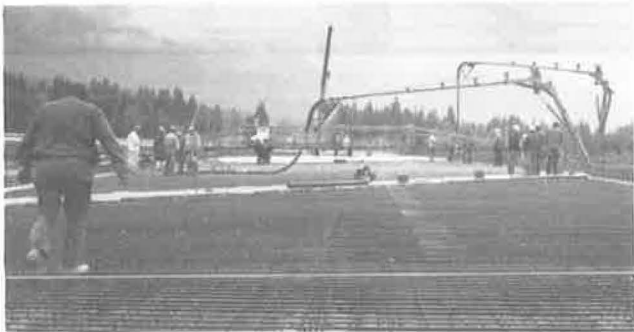
Figure 12. Bridge deck pour in operation: concrete pump in foreground placing standard class AX concrete and pump in background placing wax-bead concrete overlay.
