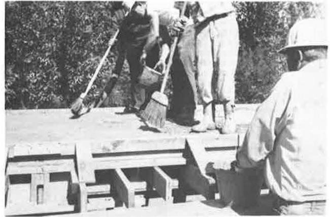
Figure 8. Grout slurry being broomed into concrete surface as a bonding aid.
