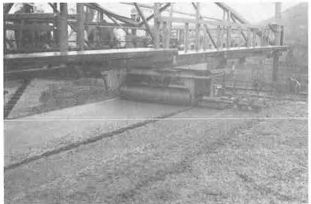
Figure 14. Bidwell finishing machine in operation with vibrating pad located between rollers and strike-off auger.
