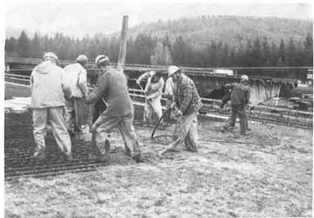
Figure 13. Lower course of conventional concrete being raked off at level of top mat of reinforcing steel after placement and consolidation by internal vibration.
