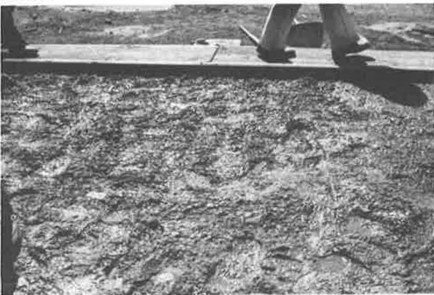
Figure 7. Texture of surface of first concrete course for test slab 3.
