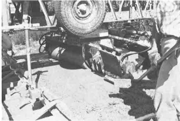
Figure 5. Gomaco 350 finishing machine in operation with strike-off auger positioned between vibrating pad and rollers.
