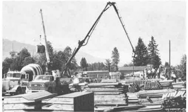
Figure 9. Thompson 10.2-cm (4-in) piston-type concrete pump placing concrete for test slabs.
