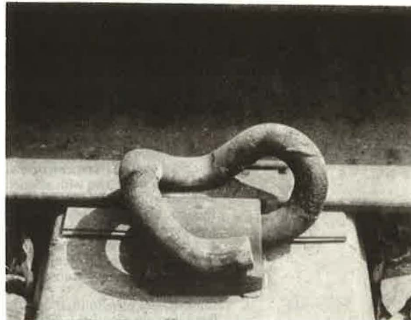
Figure 6. Rail fastener on concrete tie.
