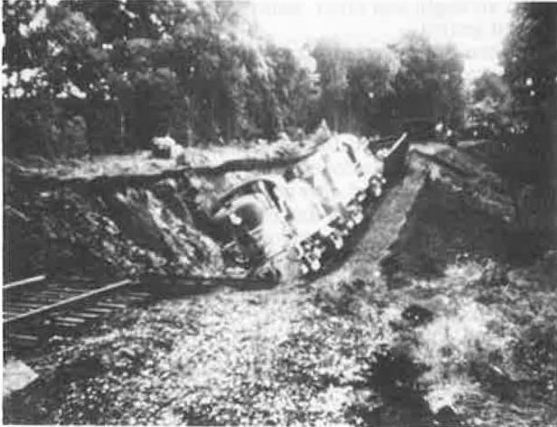
Figure 4. Embankment failure: Spar Mill Bay.
