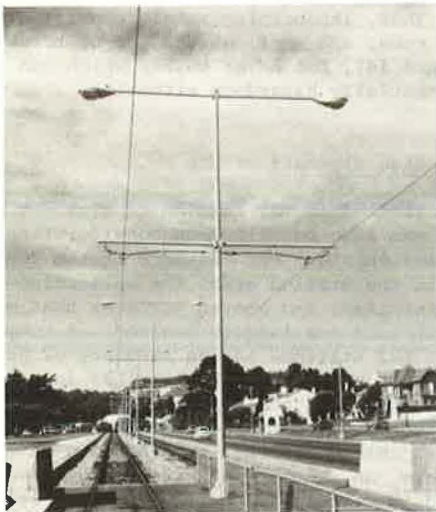
Figure 3. Coordinated, Center pole design--San Francisco.
