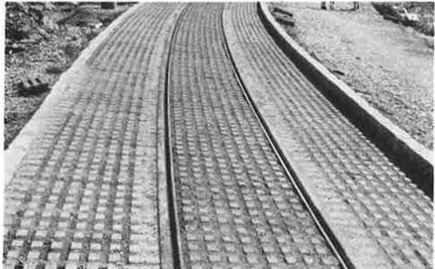
Figure 10. Track in lawn under construction--Linz.
