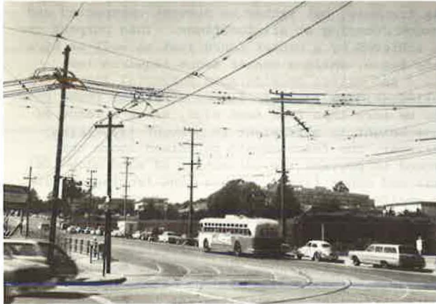
Figure 1. Overhead Clutter. A mix of overhead feeder cables, utilities, and wires for LRT and Trolley buses.
