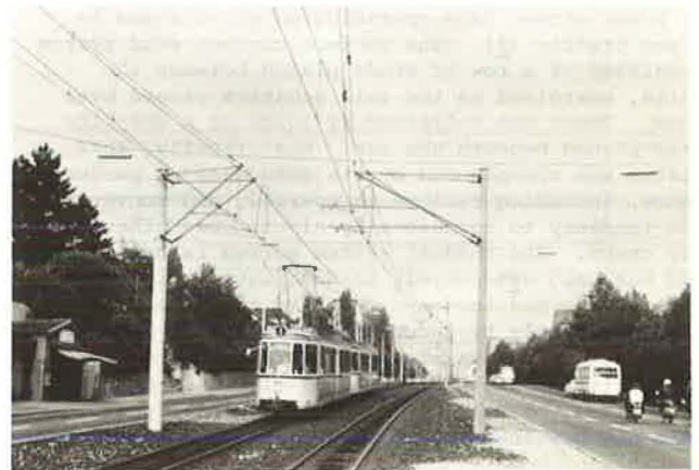
Figure 2. Uncoordinated, side pole design, with independent street lighting--Stuttgart.
