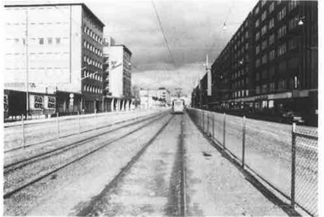
Figure 12. Side fencing where center fencing could suffice.
