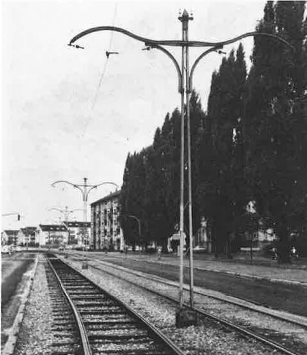
Figure 10. Track in lawn under construction--Linz.
