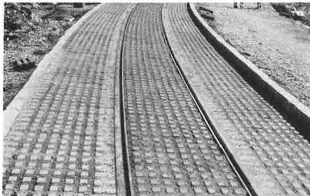
Figure 10. Track in lawn under construction--Linz.
