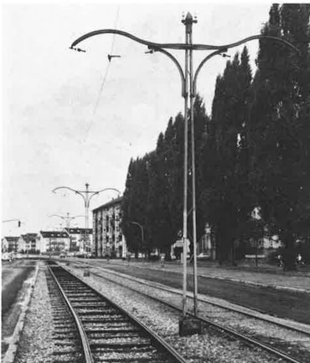
Figure 10. Track in lawn under construction--Linz.
