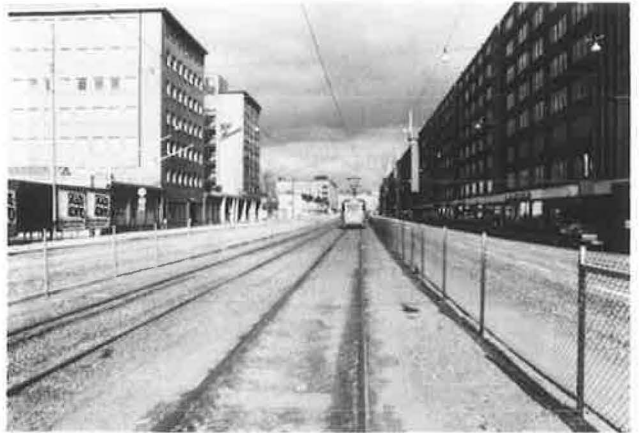
Figure 12. Side fencing where center fencing could suffice.
