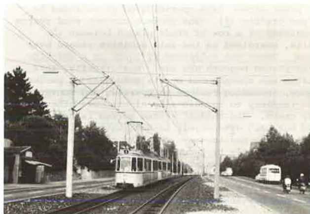
Figure 2. Uncoordinated, side pole design, with independent street lighting--Stuttgart.
