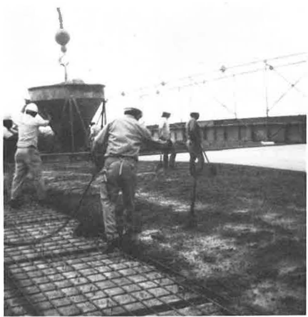
Figure 11. Concrete placement.
