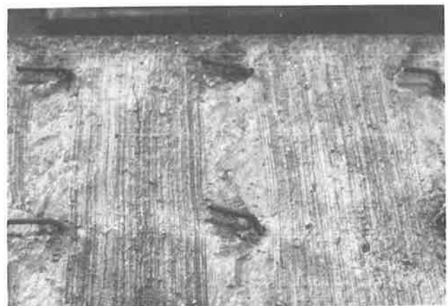
Figure 5. "Z" Bars were difficult to place.
