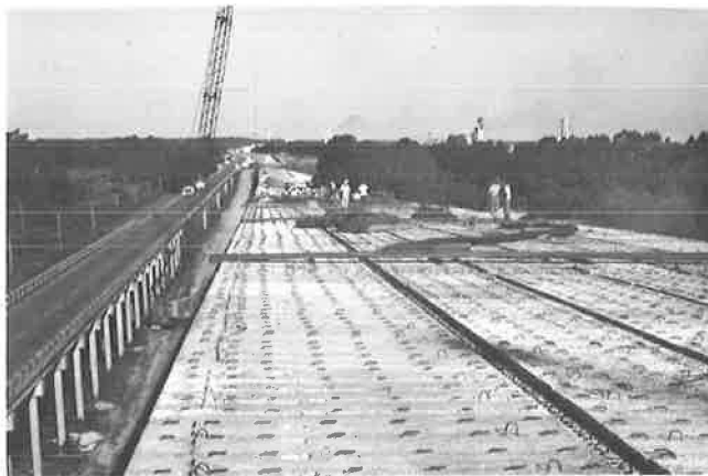
Figure 2. Trinity River Bridge near Trinidad.
