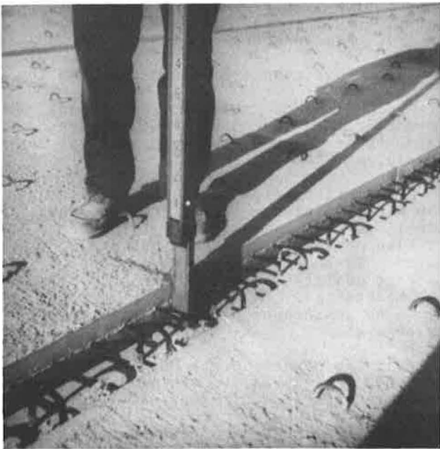
Figure 10. Grading the deck after erection of panels.
