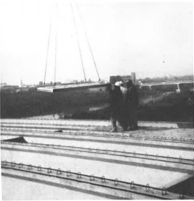
Figure 9. Panels being placed on fiberboard strips.
