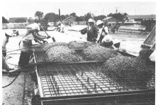
Figure 6. "U" Bars with external vibration are better.
