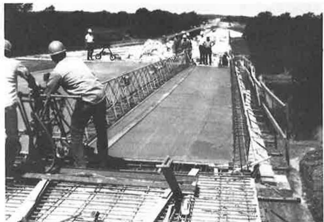
Figure 12. Concrete finishing.
