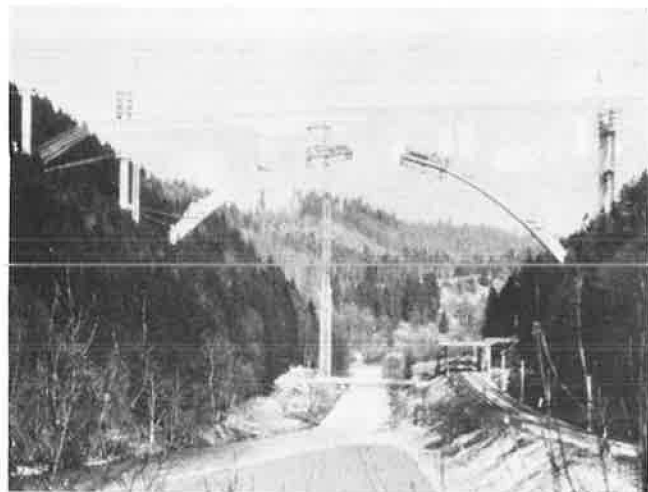
Figure 24. Rottweil-Neckarburg arch bridge.
