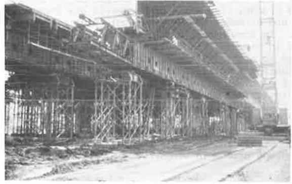
Figure 7. Ground supported form carrier, Rheinbrücke-Düsseldorf-Flehe.
