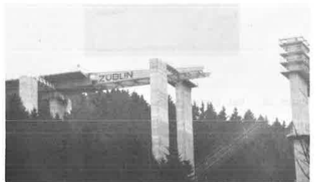
Figure 26. Launching deck on Rottweil-Neckarburg arch bridge.
