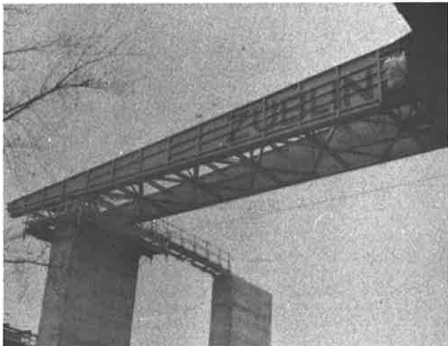
Figure 27. Closeup of launching nose Rottweil-Neckarburg arch bridge.
