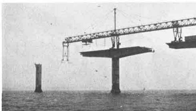
Figure 3. Launching girder, Sallingsund Bridge
