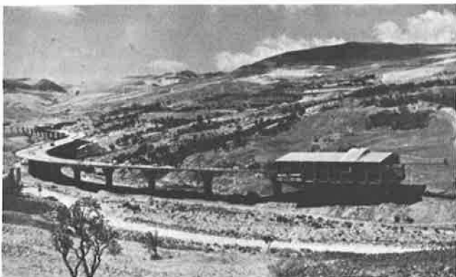
Figure 11. Viaduct Fichera - Sicily.
