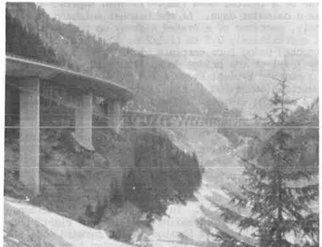
Figure 9. Brenner autobahn - Innsbrucke, Austria.
