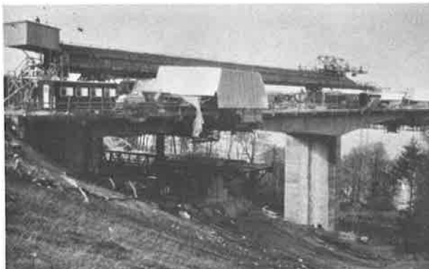
Figure 2. Launching girder, Vejle Fjord Bridge
