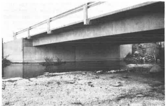
Figure 4. Bridge on county road in Washington with precast abutment and wingwalls.
