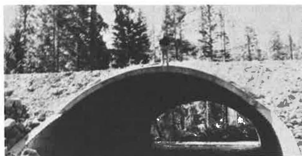
Figure 2. Horizontal arch-shaped culvert with 12 m (40 ft.) span.
