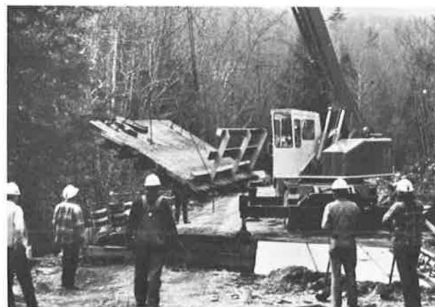
Figure 2. Precast slabs replace substandard steel stringer-timber deck superstructure.
