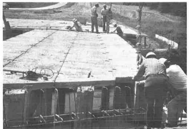
Figure 5. T-beam is placed in position.
