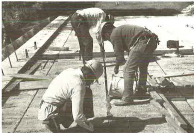
Figure 7. Nonshrinking cement paste is placed between adjacent T-beams.
