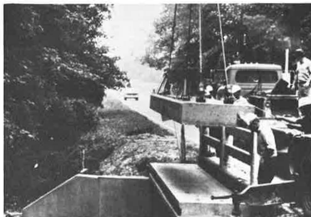
Figure 1. Precast slabs used to widen bridge.
