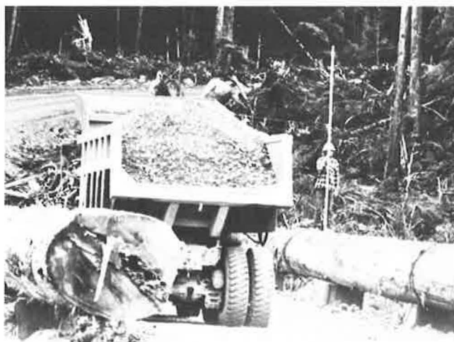
range of log stringer bridges. The fourth bridge failed during testing.
