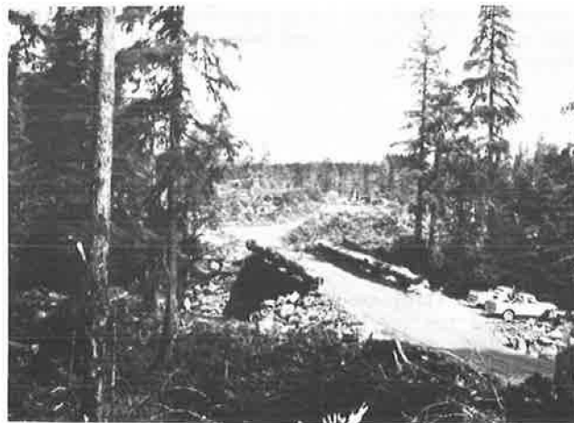
Figure 1. Native log stringer bridge in southeast Alaska: Span--28 m (92 ft); Capacity--72.5 Mg (80 tons).
